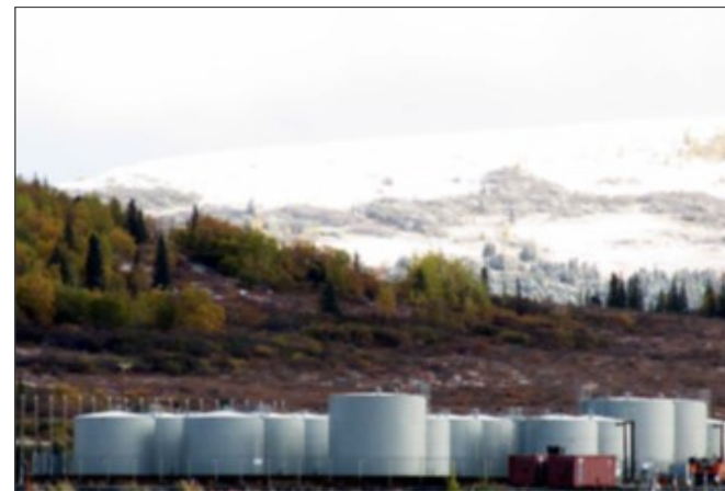
Unalakleet tank farm.
